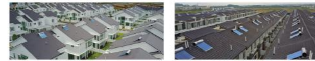
Semi-D Houses Project at Bandar Sri Sendayan by Matrix Concept Berhad 64 units 60 gal (model S-60) Solarwave
