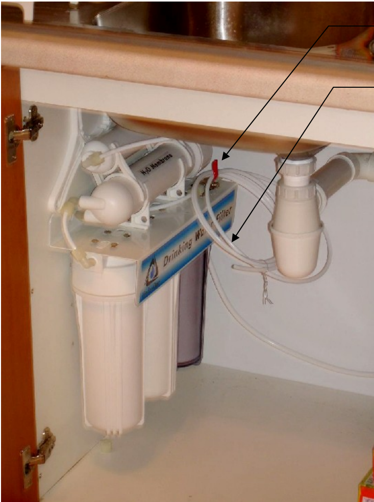
Image B – Installed Unit under sink
